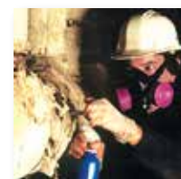
LEAD & ASBESTOS REMEDIATION
