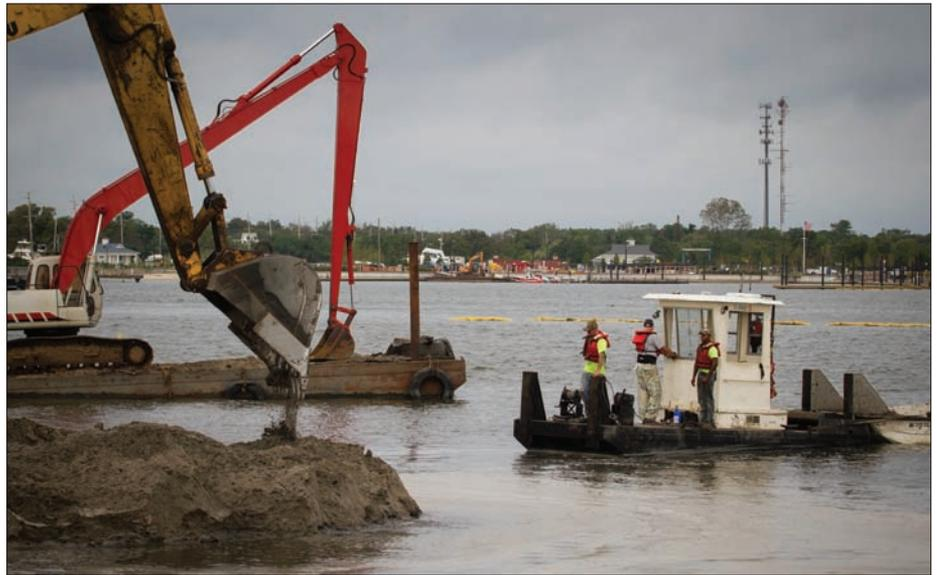
Cranes dredge New Jersey's Barnegat Bay to clear out sand and debris deposited during Superstorm Sandy. As of December 2013, the state had dredged more than 450,000-yd<sup>3</sup> from its waterways and is developing a long-term program for maintaining state channels in the future. FEMA PHOTO BY ROSANNA ARIAS
